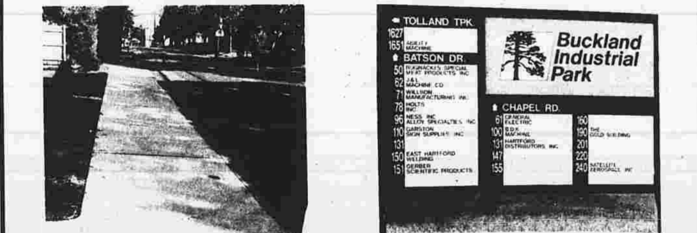
Miles of Sidewalk and Curb Repairs Underway
