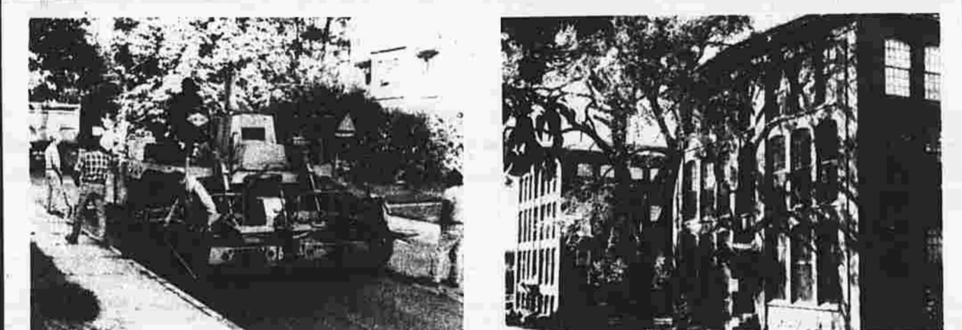
Miles of Paving Underway on Manchester Roads
